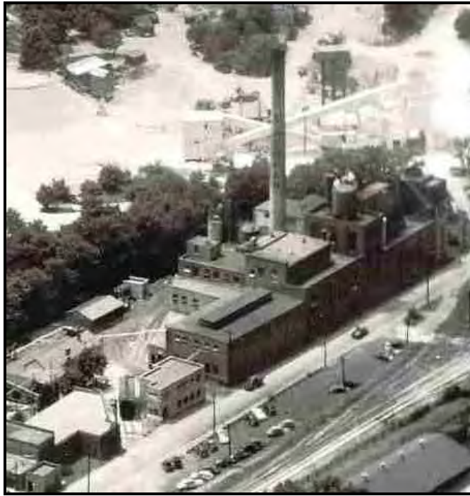
Enlargement of Distillery
